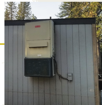
Inadequate ventilation systems need to be replaced
