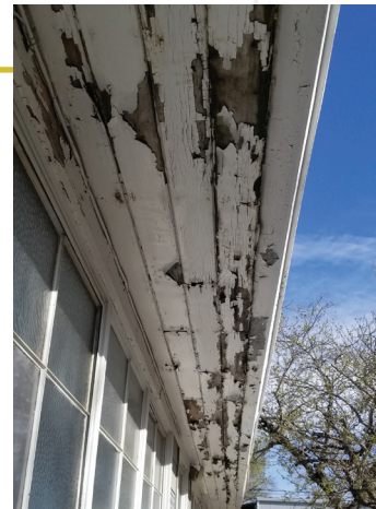
Leaky roofs must be repaired
